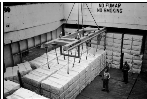
Progress over the years. 20 ton drop stow loads
